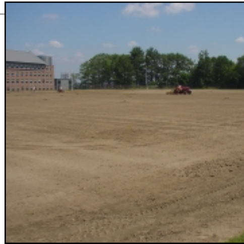
Preparing for laser grading
