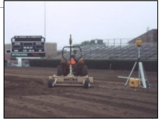
Establishing final grade
